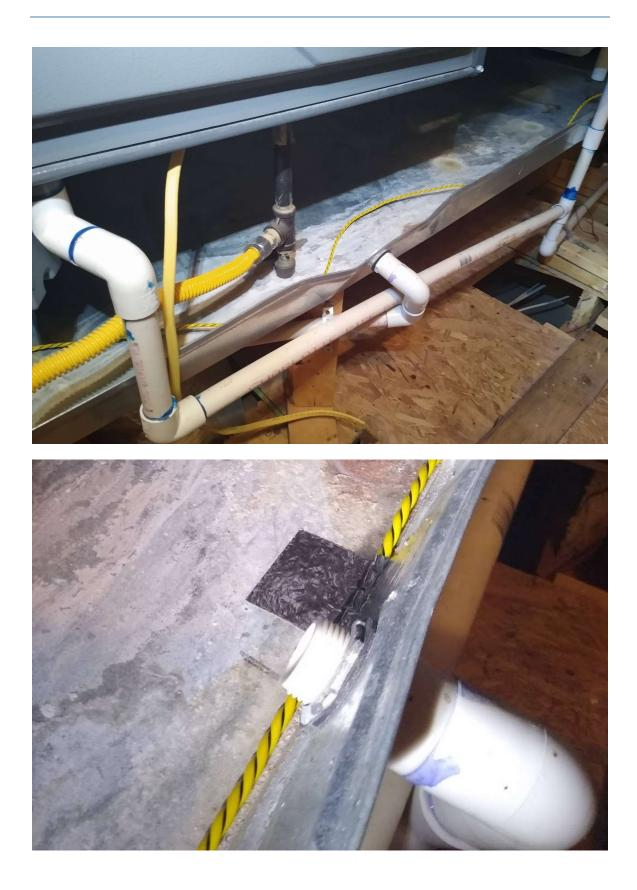
The two pictures below show the final location of the SN400 sensor node with all the sensor wires installed. It is attached to the air conditioner evaporator.
