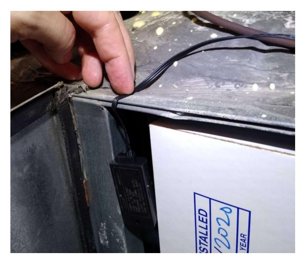
Simply close the air filter door, and for this installation, the inlet temperature/humidity sensor install is finished. After this probe was setup, the filter door was checked, while the unit was running, to see if there was any escaping air around the door seal. No escaping airflow could be detected.
