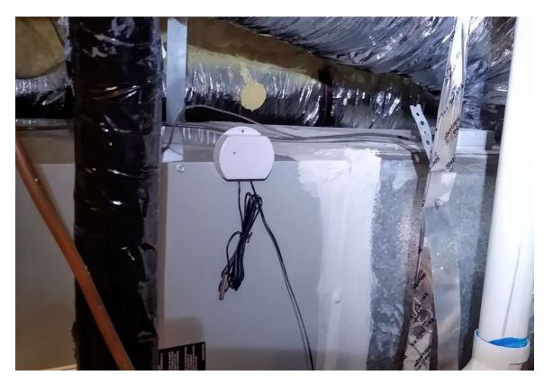
The SN400 sensor node is attached near the middle of the AC unit so probes can be fitted to both the input and output baffles. In addition, the water break sensor is positioned under the AC unit in the drip pan. In the picture, the node is held in place with integral mounting magnets.
