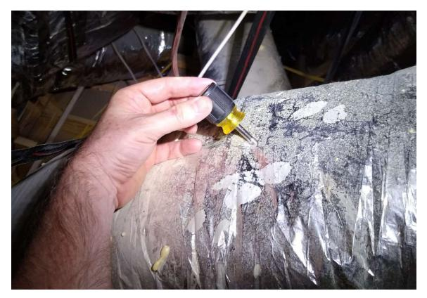
Insert the temperature probe though the hole so it is just inside the duct, and then carefully tape in place with the foil tape so no air will leak out of the duct. Use about three overlapping layers to prevent air leakage. This is done for both output baffles of the air-conditioner, as both upstairs and downstairs output temperatures are measured independently. Refer to the two pictures below.
